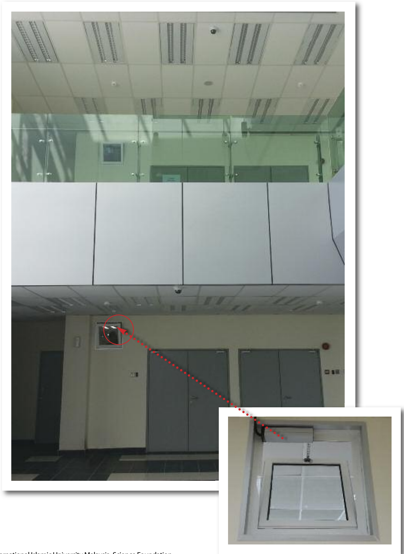
International Islamic University Malaysia, Science Foundation Centre, Phase 2, Gambang, Pahang, Malaysia.
